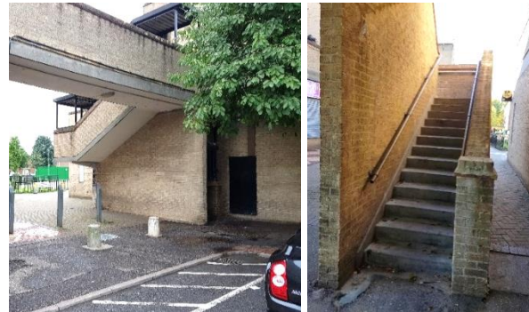
Stairs to flats before and after the corrugated roofing was removed
