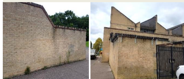
The flank wall before and after the anti-climb topping was fitted
