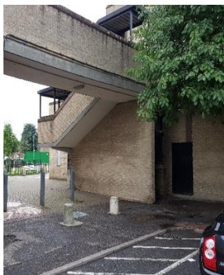
Stairs to flats with the corrugated roofing
