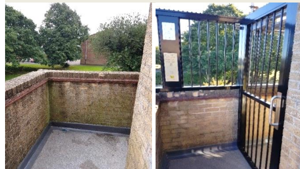
1 st floor balcony before and after access control gates were installed
